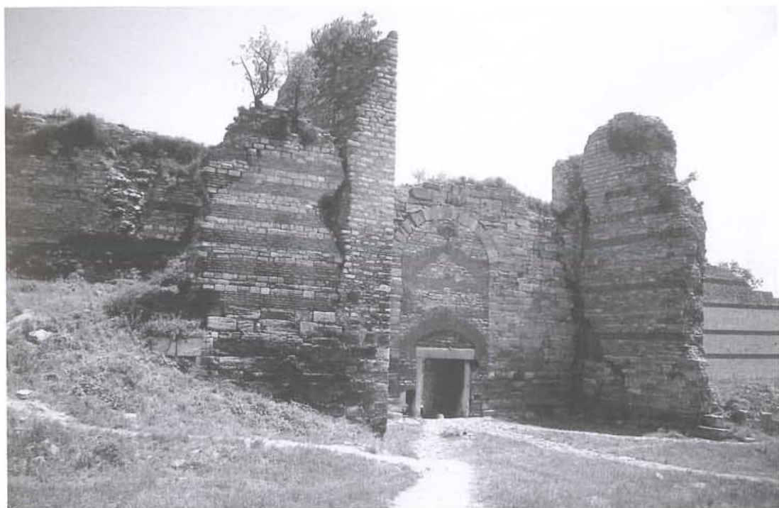
Plate 25 Outer Wall about Pempton
